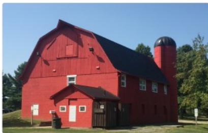
Above: The iconic Red Barn at Grand Vue Park.
